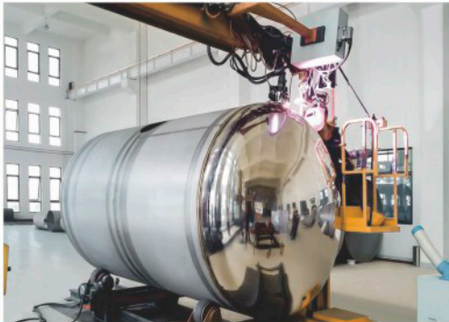
等离子自动环焊 Plasma automatic girth welding
